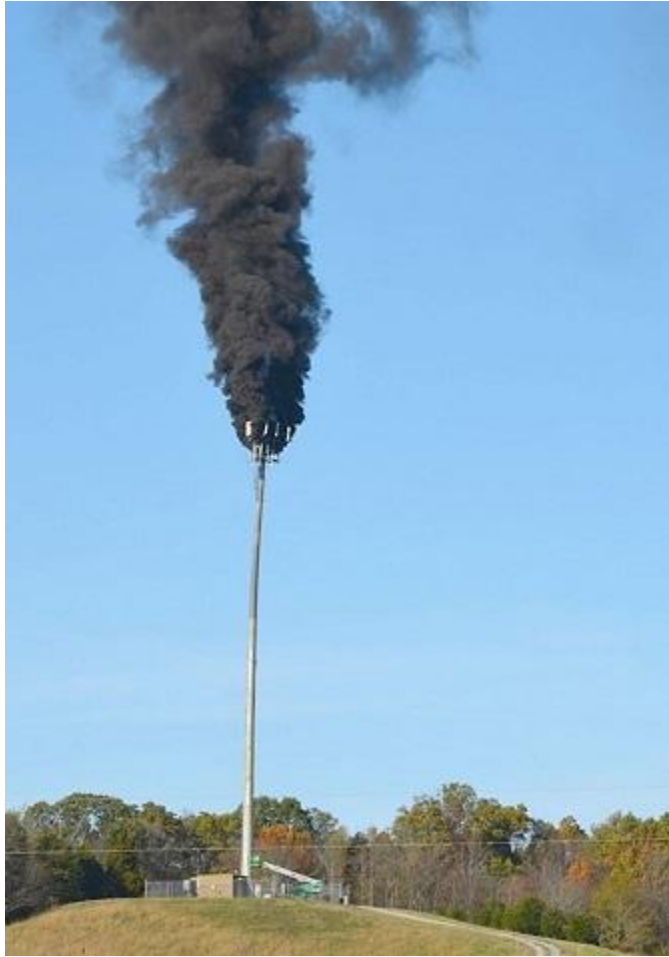
Cell tower fire caused by improper welding. Greeneville, TN, Nov 4, 2014 https://www.greenevillesun.com/xml/nitf/flames-damage-verizon-wireless-tower/article_1619f00e-5383-530a-a69e-0dbd2acc3c6a.html Photo credit: Kristen Buckles
