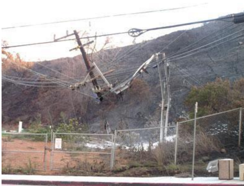
Malibu Canyon fire, 2007 Overburdened with weighty telecom gear, the pole collapsed. 14 houses burned.
