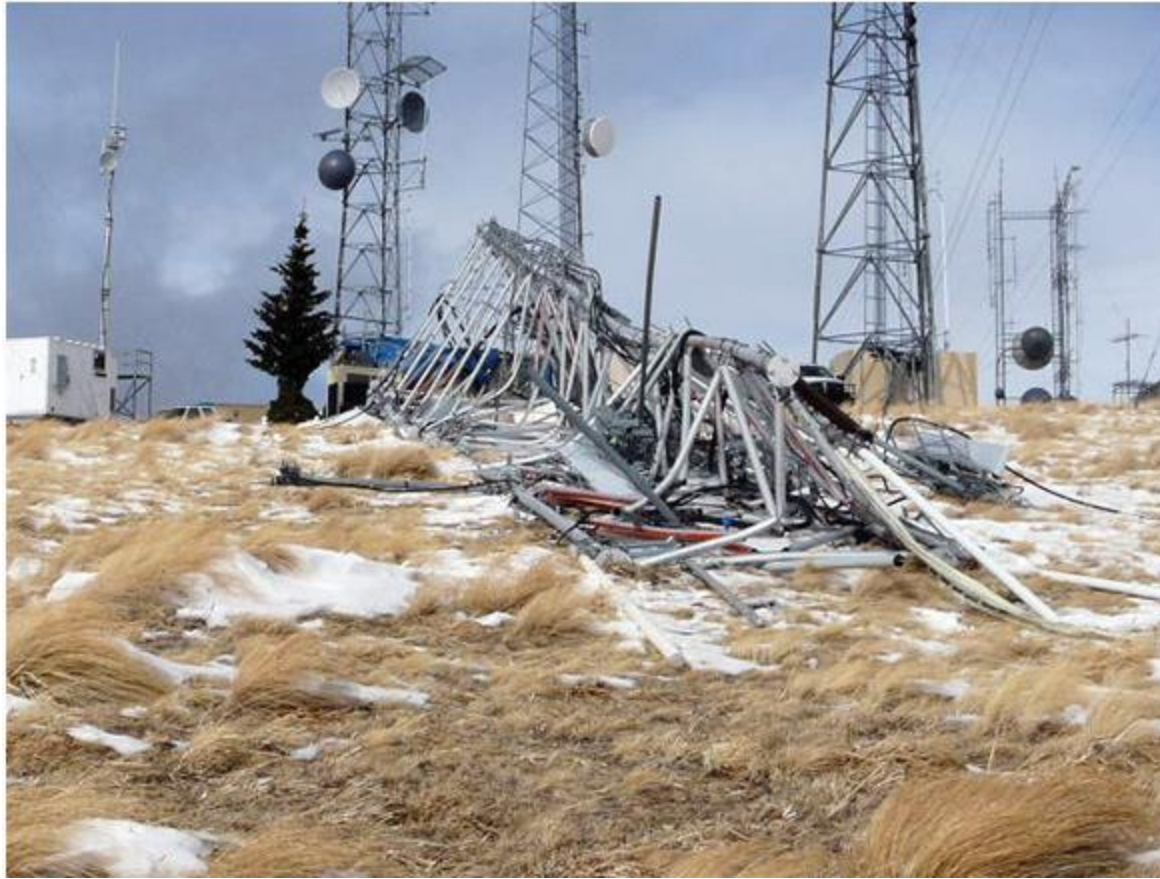
Cell tower collapses in high winds. Ruidoso, NM, Dec 18, 2009 http://wirelessestimator.com/content/articles /?pagename=Cell_Tower_News_12.09 Photo credit: Steve Kitchens
